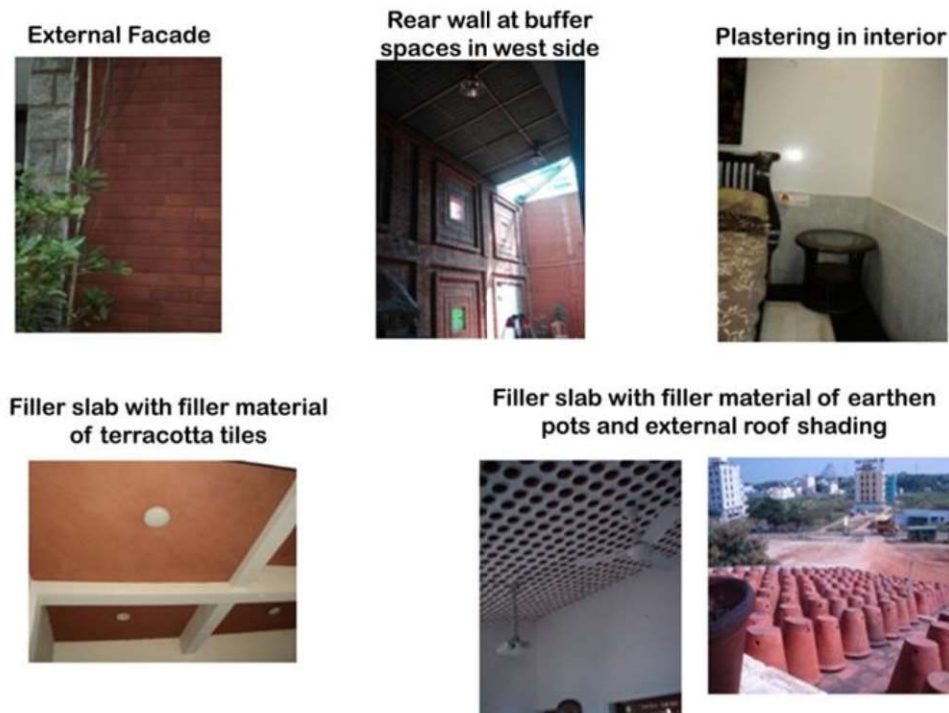
Figure 7: Envelope materials used in contemporary house with sustainable construction techniques
